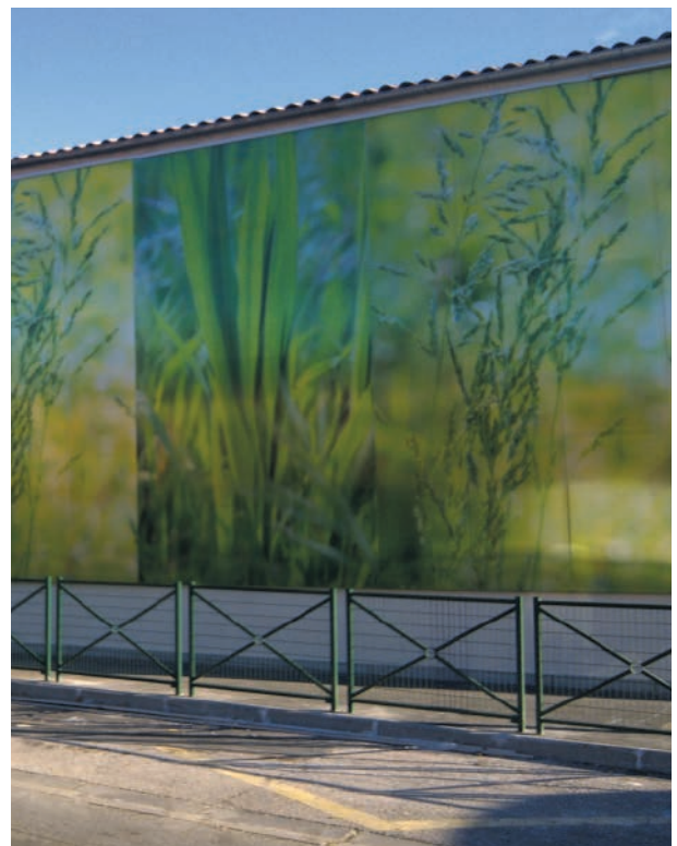
Santoni School, La Garde, France Glazing: Danpalon® Printed, 16mm Architect: La Garde, Becker Sylvie
