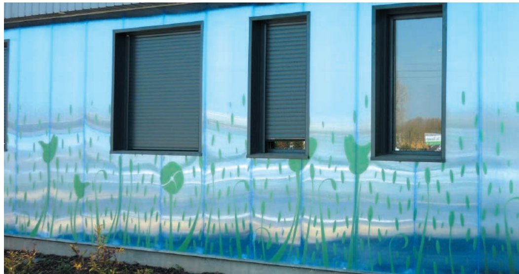
Liberty Creche, Le Petit Quevilly, France Glazing: Danpalon® Printed, 16mm Architect: Gérard Bourdon
