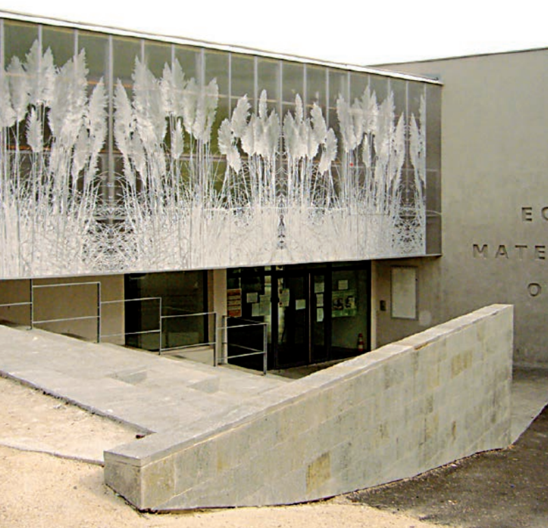
Oddo Nursery School, Marseille, France Glazing: Danpalon® Printed, 16mm Architect: Camille Richard Lenoble
