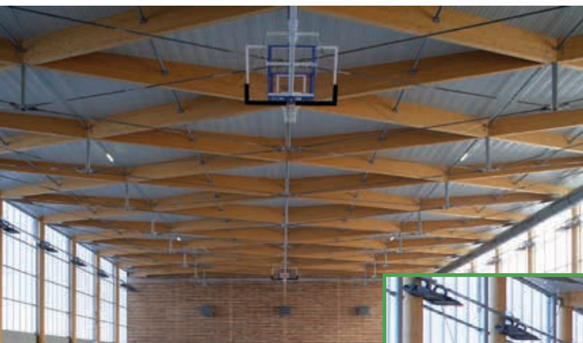
Sports Hall, France | Controlite® Architect: Gremillet
